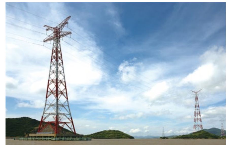
Heaviest tower Zhoushan: 7,280 ton
