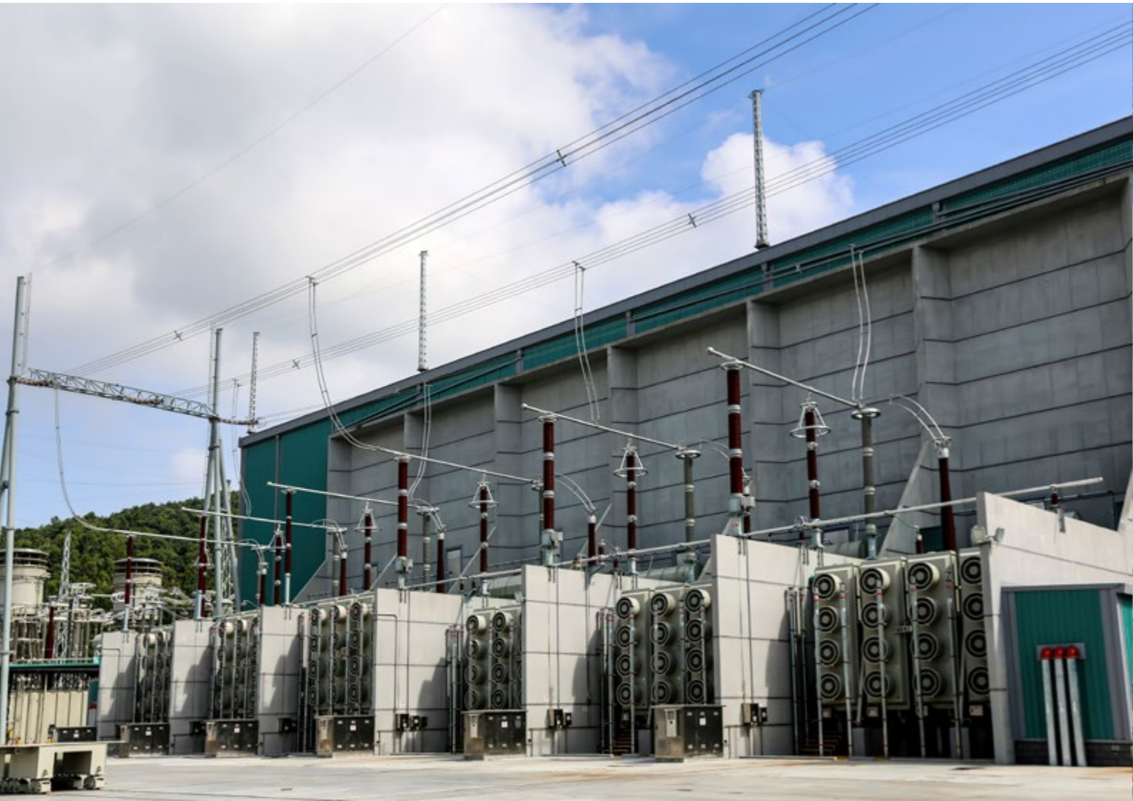
▲ ±800kV Converter transformer for UHV DC from Lingzhou-Shaoxing Transmission Line Project, China
